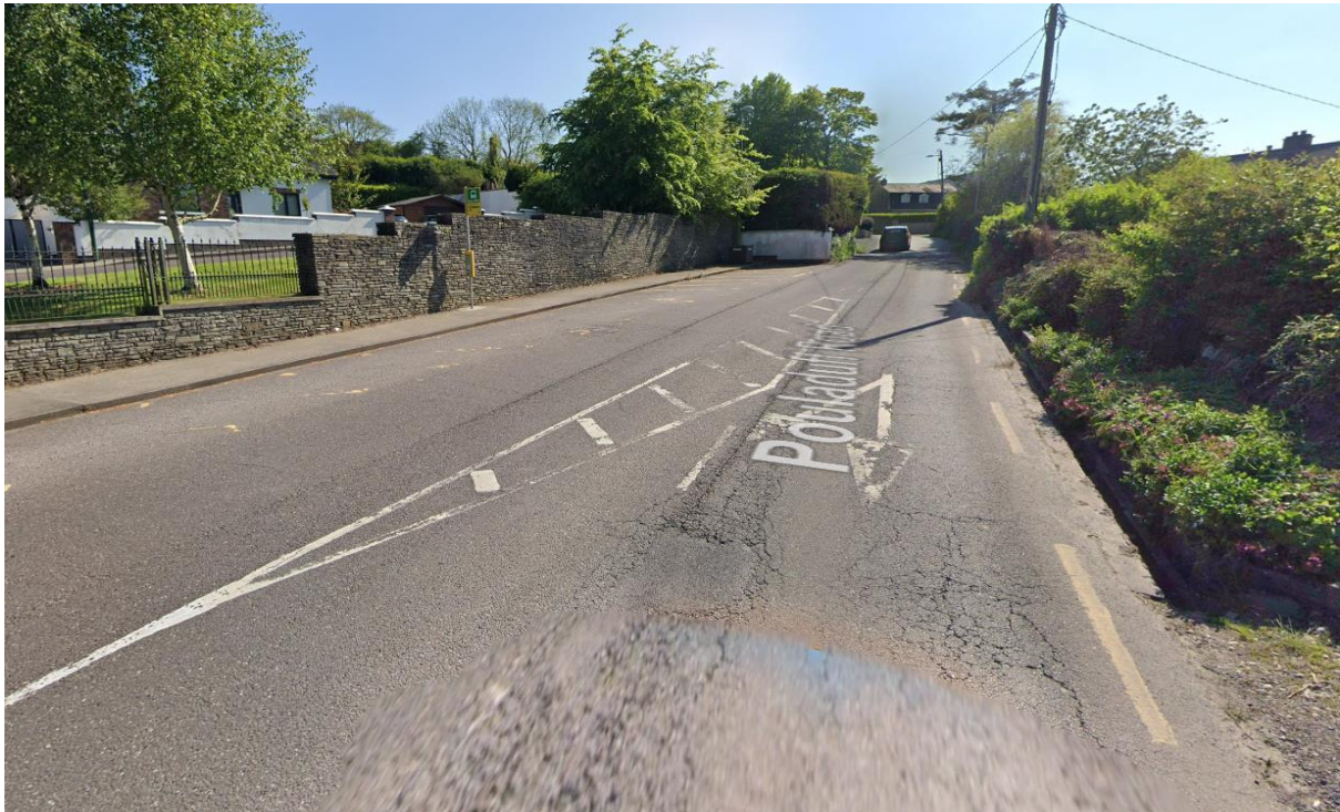
Area for Night works.
