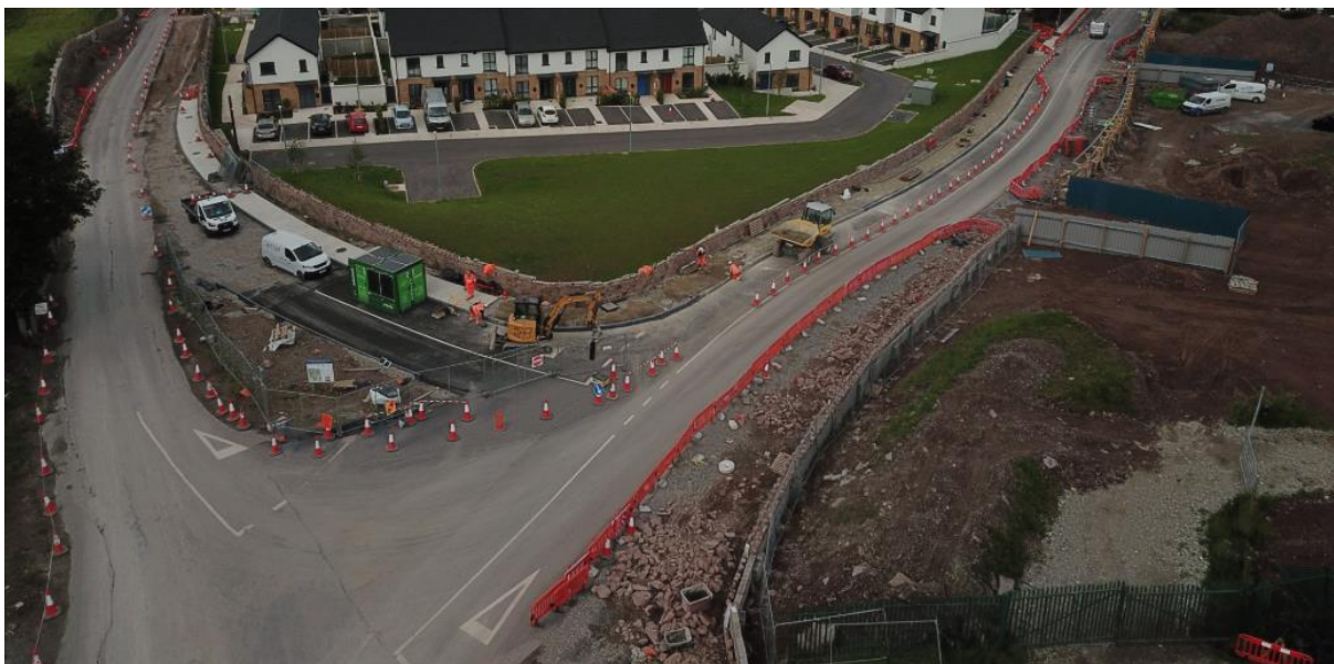
New junction layout under construction.
