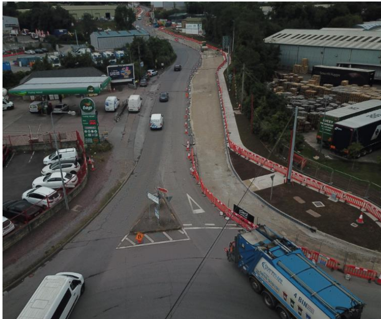
Road construction and new footpath leading into the Roundabout at Cork Builders Providers
