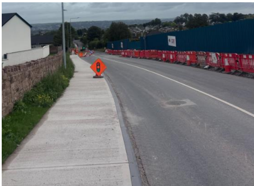
Surfacing crews working at Mathew Hill estate.
