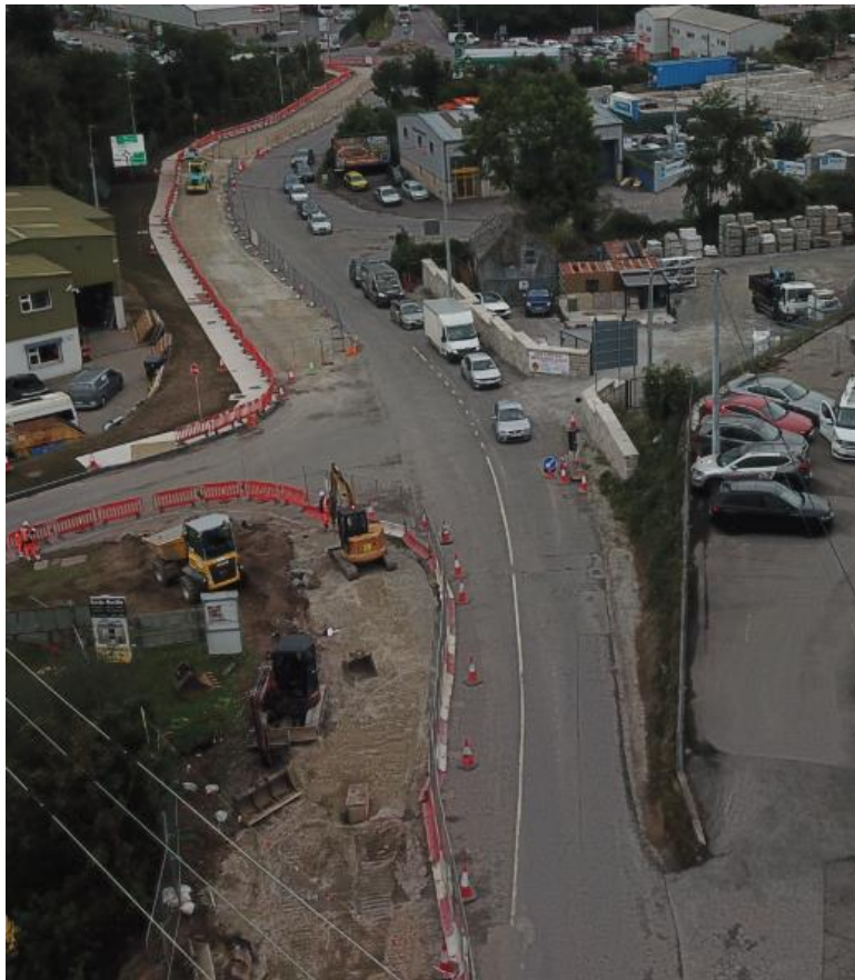
Road Widening Works at Forge Hill Junction
